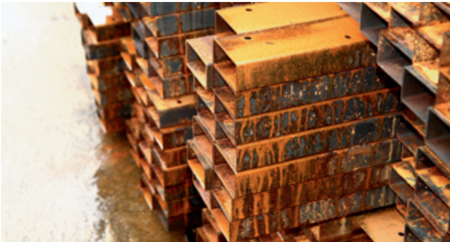
Fig. 4: Corrosion of steel components.
