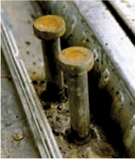
Figure 5: X-HVB shear connector in rehabilitation
