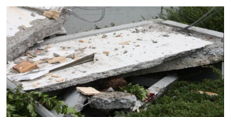
Balcony crash due to insufficient rebar reinforcement
